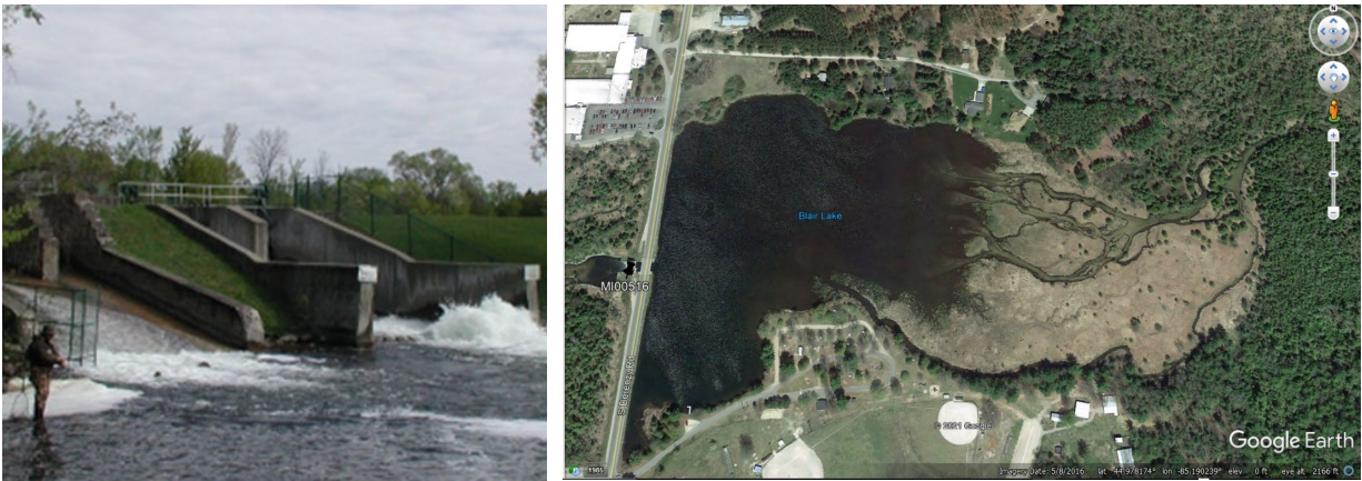
Figure 28. Photograph of the Cedar River Dam Spillway, Extensive Reservoir Deposition is Apparent on the East Side of the Cedar River Dam Reservoir, (MI00516), Built in 1890, Elk River Watershed (13) (Aerial Photograph, Google Earth Pro, 2021)
